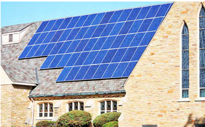
Church with solar panels.
